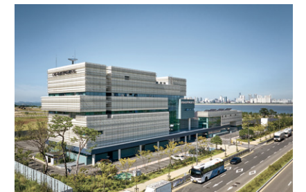
Research Building 3 (Unmanned Mobility Laboratory)
