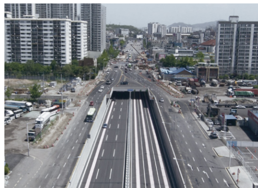
Expressway between Incheon and Gimpo PF Project
