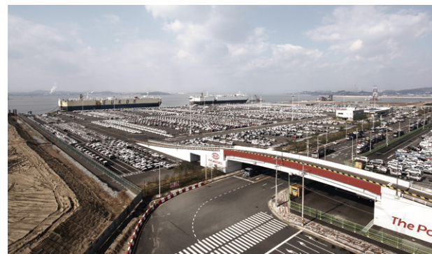
Vehicle-only quay for Pyeongtaek Port (Berth nos. 9 and 10)
