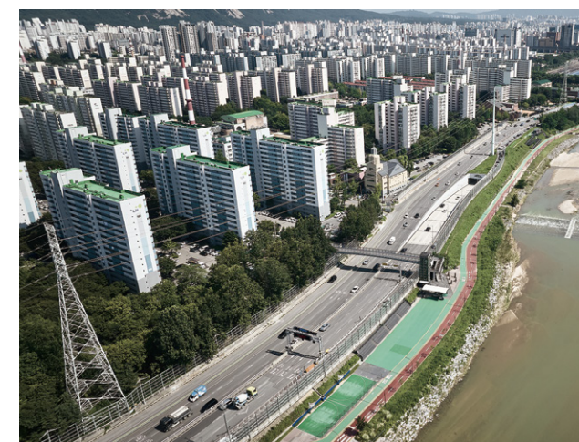
Extension of Dongbu Expressway
