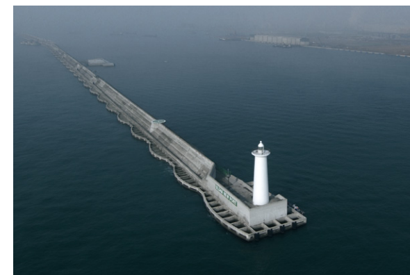
North breakwater at Ulsan New Port (Zone 2)
