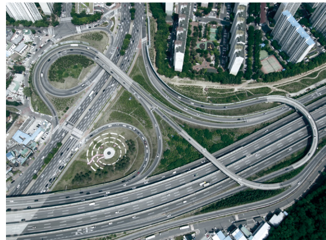
Extension of Expressway No. 451 from Seongseo to Okpo (Zone 1)
